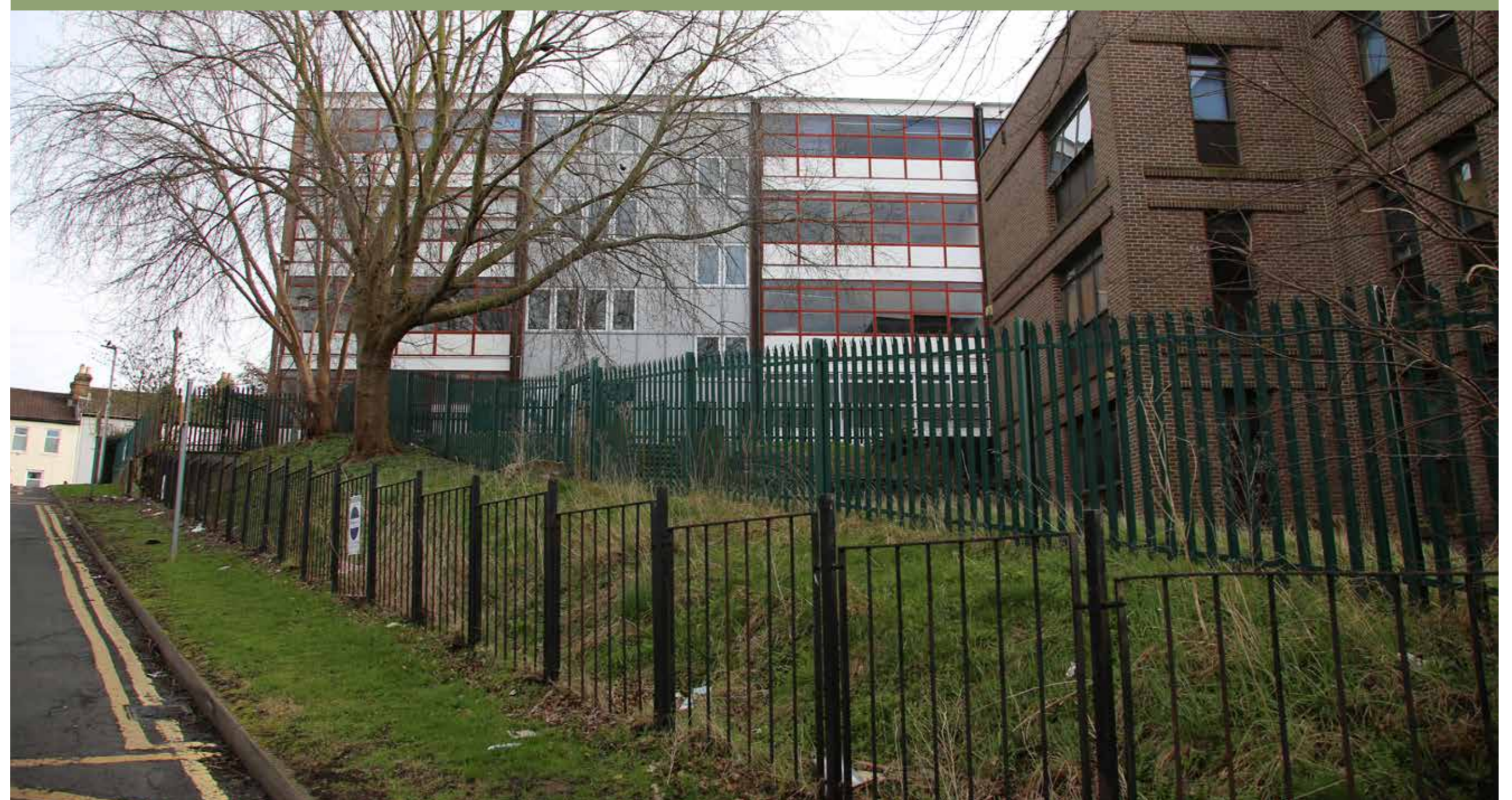
VIEW OF EXISTING SCHOOL BUILDINGS FROM CHARLES STREET
