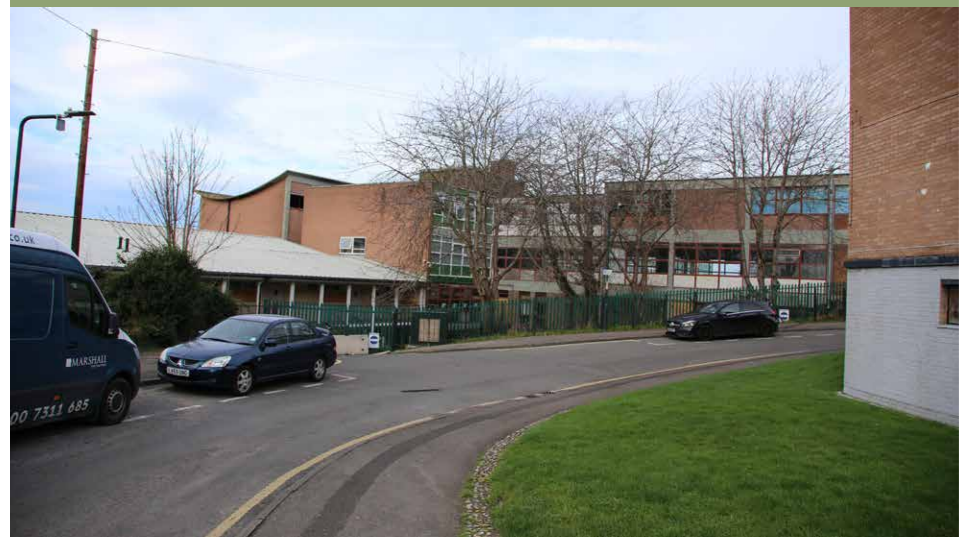
▶ VIEWS OF THE EXISTING SCHOOL BUILDINGS AND ACCESS FROM PERRY STREET
