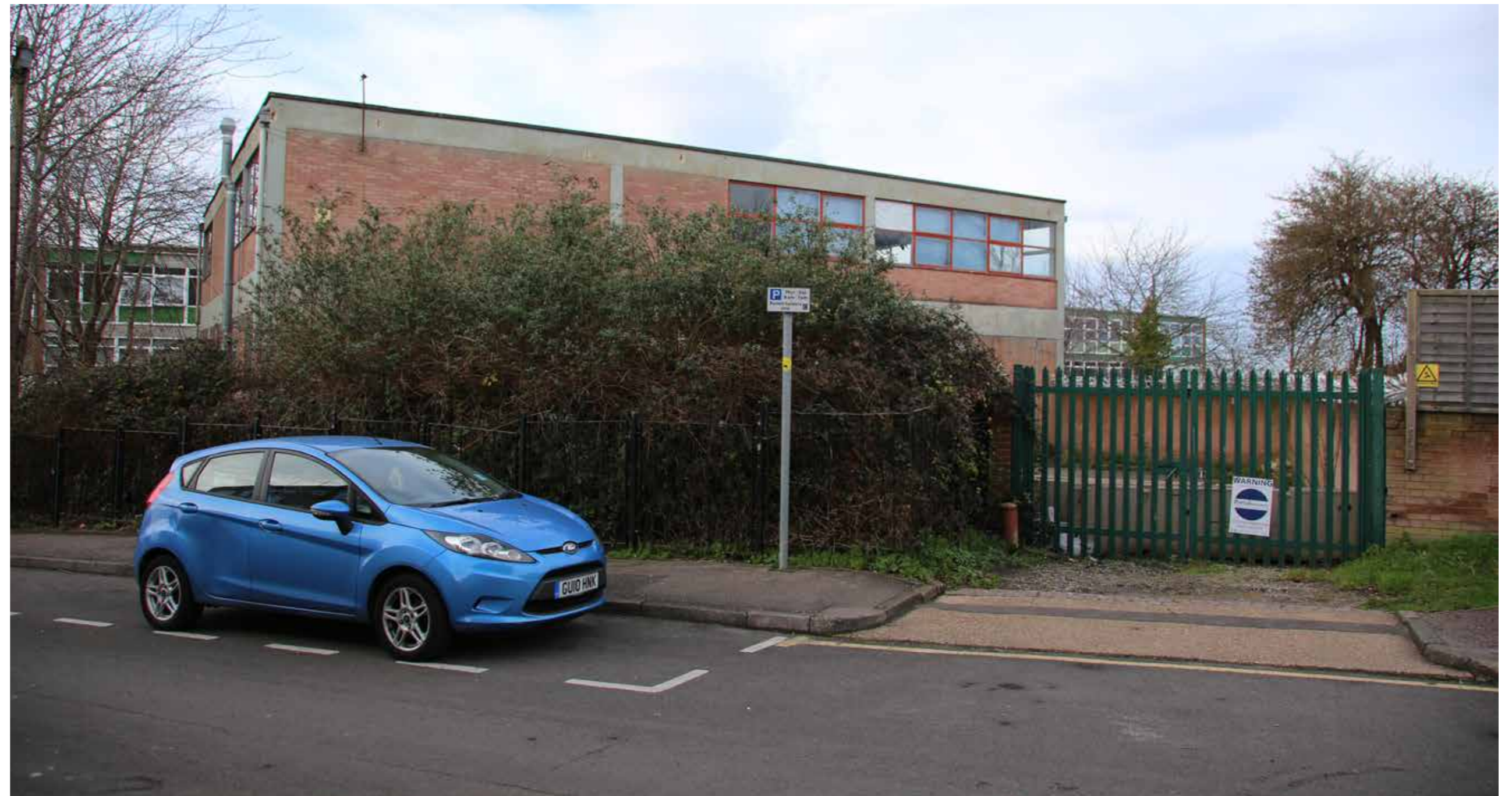
VIEW OF EXISTING ACCESS TO SCHOOL FROM PERRY STREET
